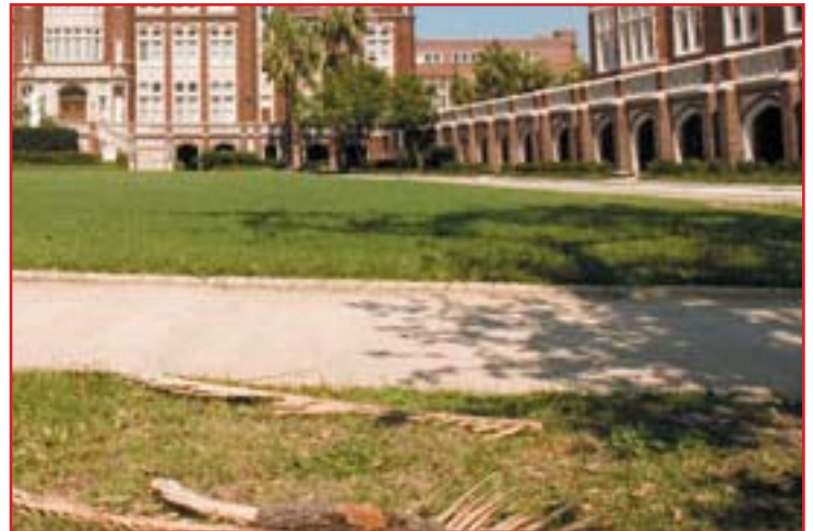
From the Loyola University New Orleans Website: 9/7/05: Loyola University is fortunate that its campus was spared significant damage from Hurricane Katrina. These photos were taken right after the storm. University Police and Physical Plant personnel stayed on campus during the storm and are currently still on campus.
